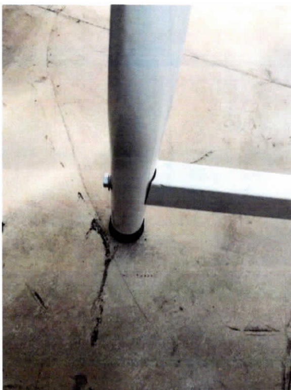
1-3: Using the bolts to connect the leg to the beam.
